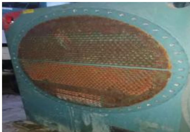
Tubes With Fouling
